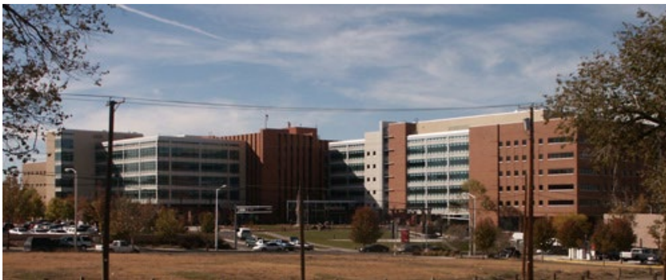
Identify the nearest emergency medical facility and develop a plan in advance to get injured workers to the facility.
